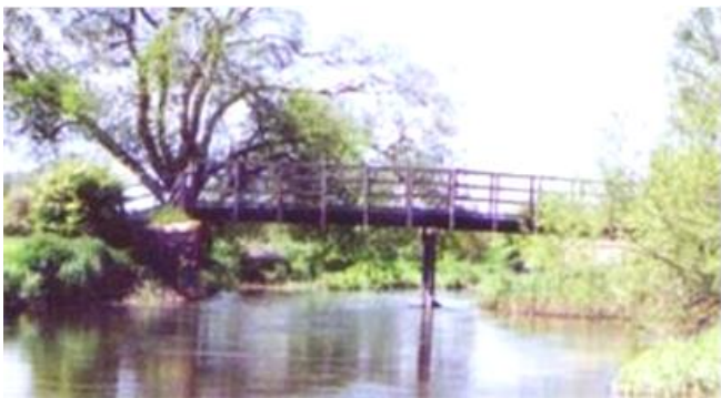
Water Eaton Bridge
