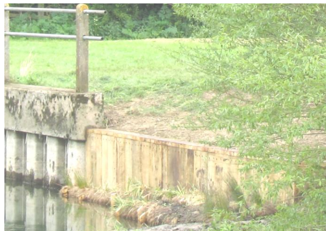
Photo 4 – Bank Protection and Coir Rolls for Water Voles
